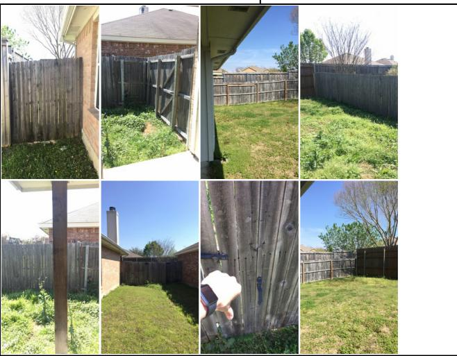
**Comments:** Grate handle needs to be reattached. Overall fence is standing; wood rotting. Would reccomend future budgeting for fence repairs.
